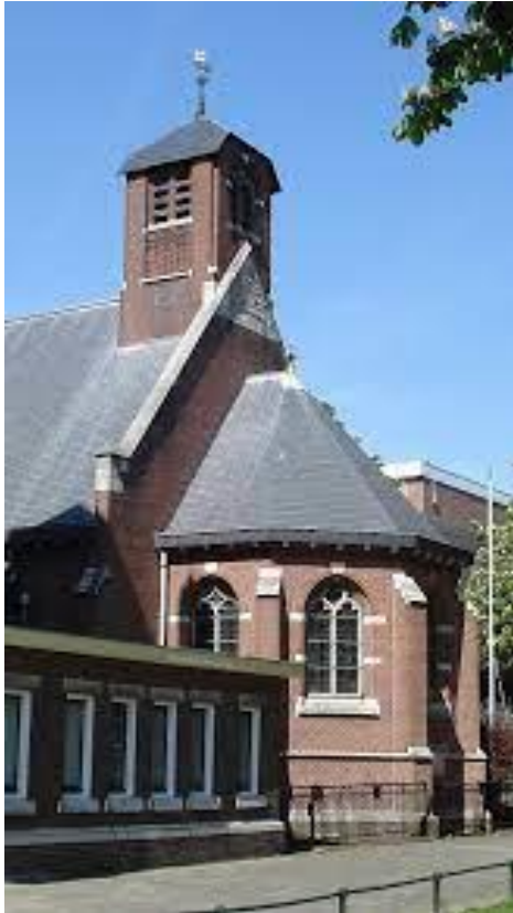
St Mary's Church Delfshaven
