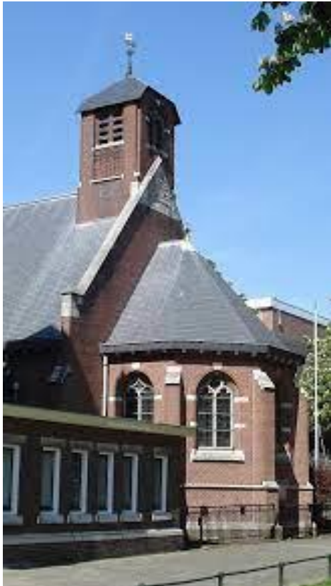
St Mary's Church Delfshaven
