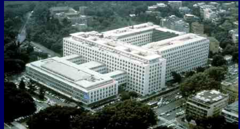
FAO building, Rome 1993 - 2000
