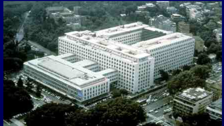
FAO building Rome
